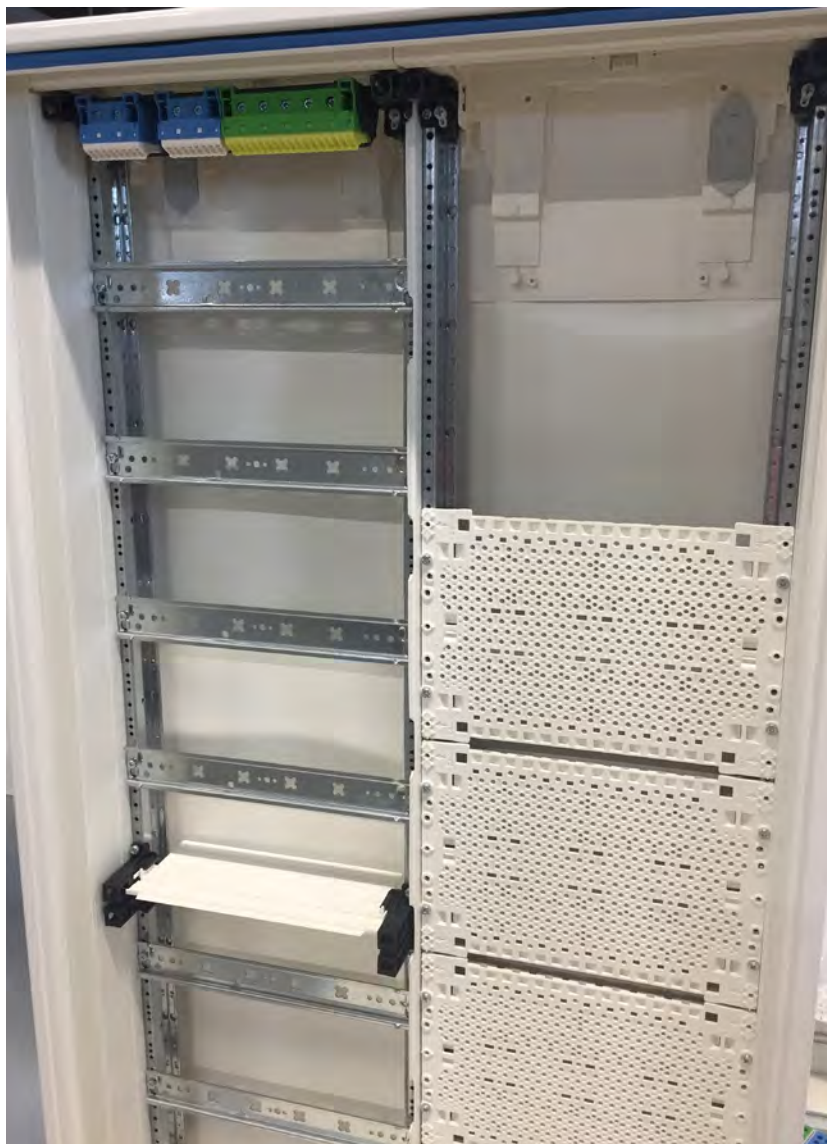
Cabinet with installed partitions
