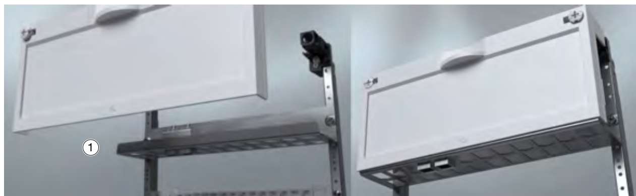
Installation of the patch panel cover with 2 fixation towers
