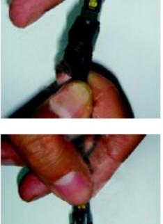
And maintaining the cable bending with right hand, push the connectiong holder forward to the end and fix the fiber.
